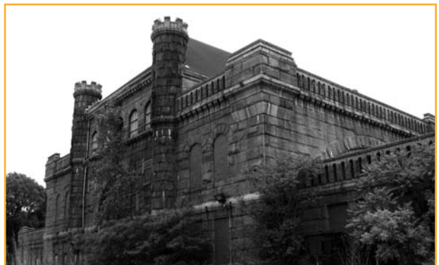
The Calf Pasture Pumping Station on Columbia Point in Dorchester was recently transferred to UMass, Boston. HBI received a grant from the National Trust for Historic Preservation to study feasible re-uses for this Romanesque Revival building that will serve the University and the surrounding community.
