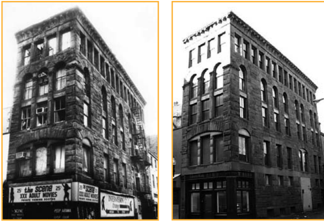
HBI's purchase and rehabilitation of the H. H. Richardson designed Hayden Building, pictured above before and after our work, helped Chinatown businesses replace adult entertainment uses in the area formerly known as "The Combat Zone."
