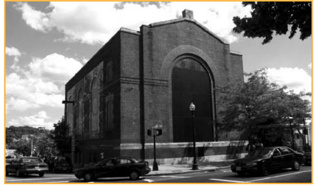
In cooperation with Roslindale Village Main Street, HBI prepared a feasibility study on the preservation and reuse of this 1911 MBTA Substation, a pivotal Roslindale Village structure.
