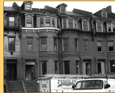
HBI's partnership with the BRA involving the structural stabilization and exterior restoration of the rowhouses at #7 & 8 Alvah Kittredge Park (the two farthest right in these "before" and "after" pictures from 1999 and 2006) enabled the rehabilitation of these two structures by their two new owner occupants while also stimulating major private investments in the other two rowhouses.
